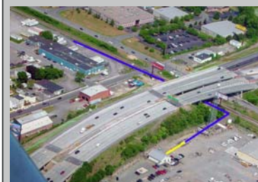
Albany, NY Aerial view of the cable project Picture owned by Superpower
