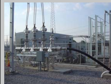
Southwire Triax Cable Termination (Southwire, 2008)
